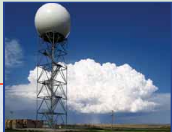
Doppler radar for measuring the velocity of wind, NOAA Photo Library, Flickr.com (Creative commons).
